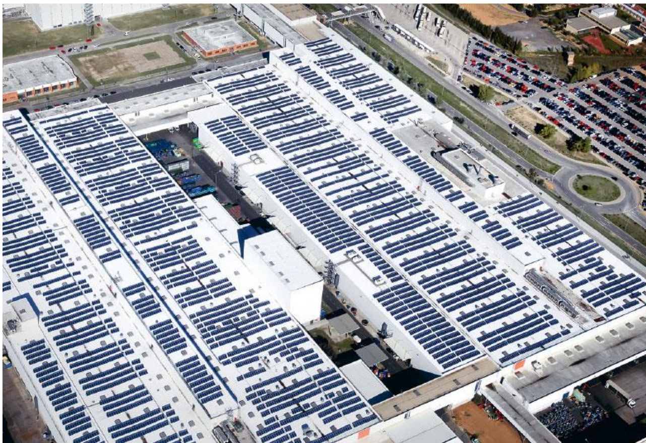
12 MW photovoltaic system SEAT car manufactory, Martorell, Spain
